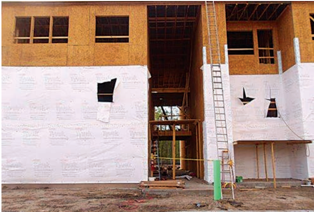
Front of building under construction
