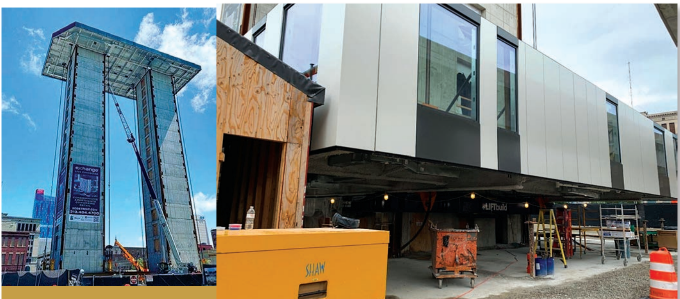
The LIFTbuild LLC. eXchange site is shown under construction in 2022.
