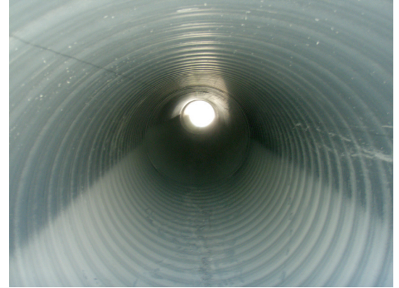
Smooth Interior Wall
