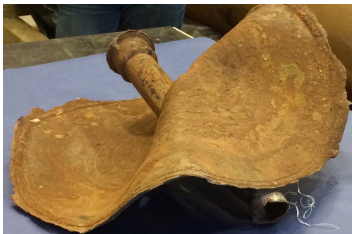
Figure 8. Close-up of bottom tank circle and portion of bottom piping showing weld seam and, outside of the seam, the thinned original bottom head “ring” material
