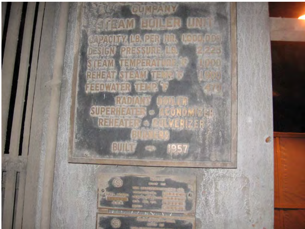
39. Boiler Dataplate
