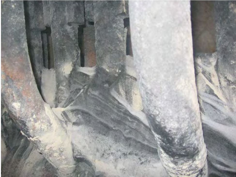
44. West side dead air space. Ash on top of header
