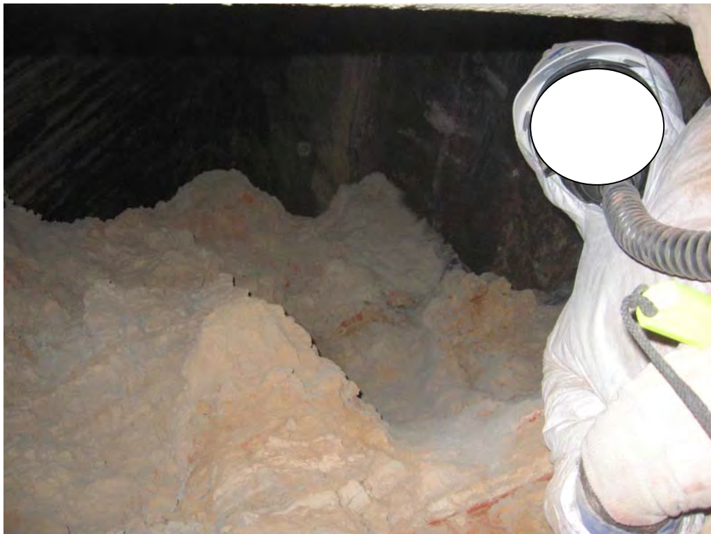
47. West side dead air space before ash is completely removed
