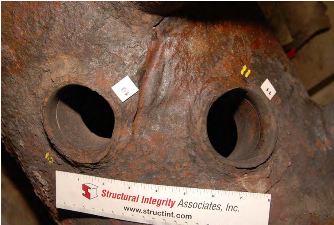
18. Close-up of header at tube 10 and 11
