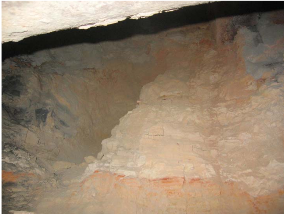
46. West side dead air space before ash is completely removed
