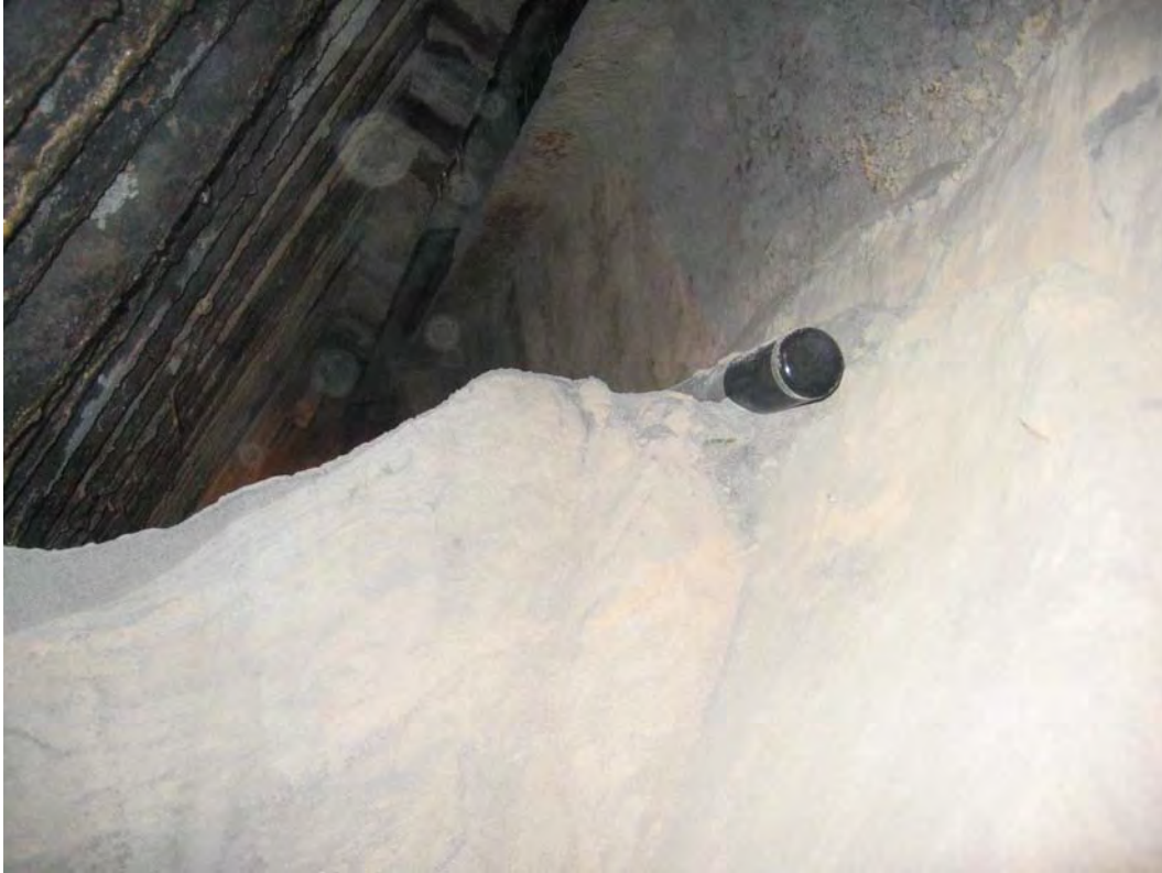
42. West side dead air space before ash is completely removed
