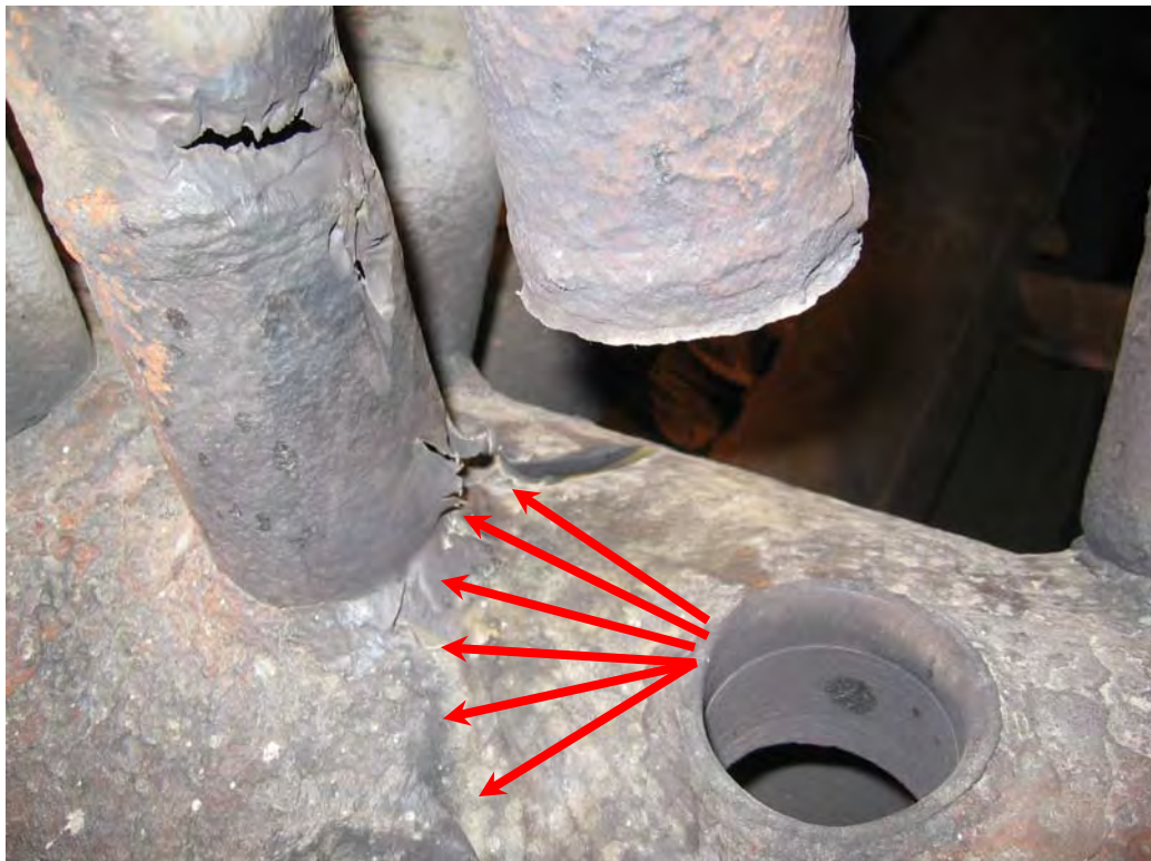
14. Close-up of header at tube 9 and 11
