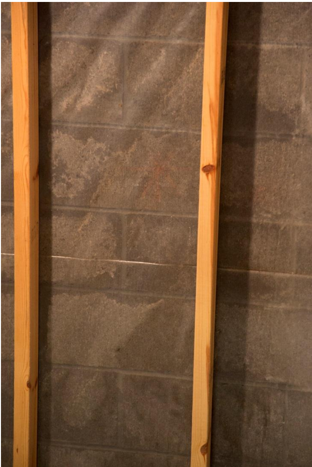
Figure B.9 Condition of an interior WSP on a masonry block wall with no interior insulation and exterior damp-proofing to grade in a well-draining sandy soil after a period of persistent rain (15 years after construction).
