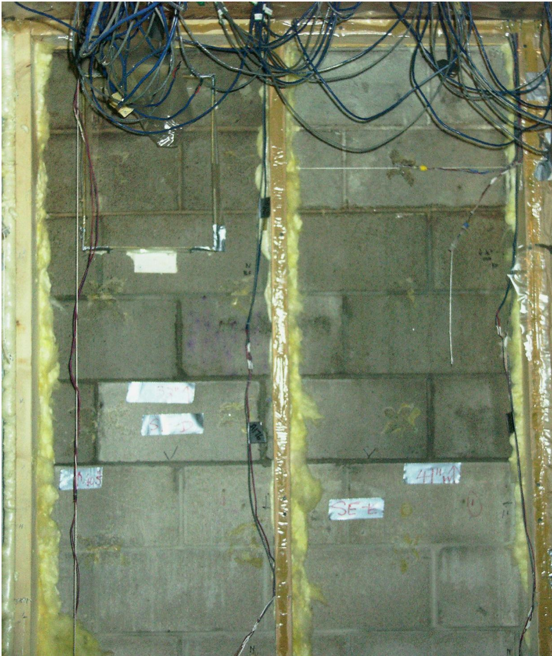
Figure B.21 Surface of the south-facing wall at tear down on 2/14/05
