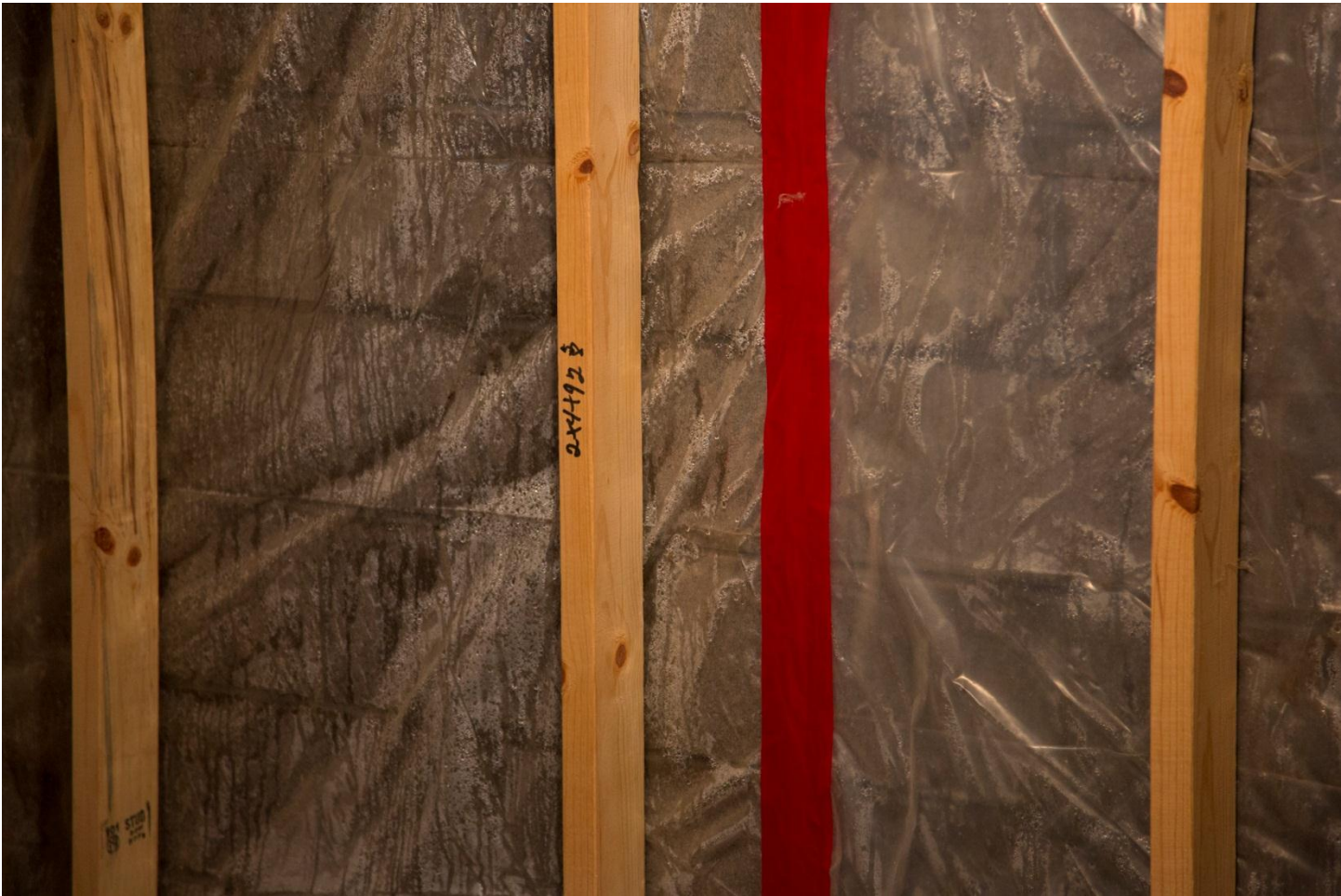
Figure B.9 Condition of an interior WSP on a masonry block wall with no interior insulation and exterior damp-proofing to grade in a well-draining sandy soil after a period of persistent rain (15 years after construction).
