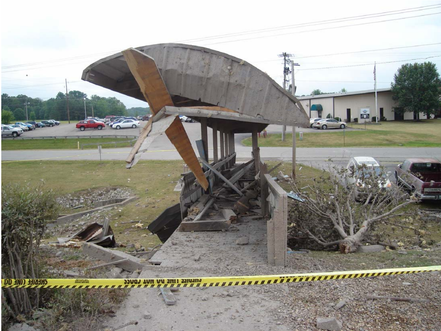
Photo #8 – View of Pedestrian Walkway Bridge
